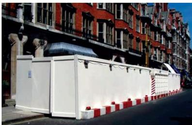
constraints were clearly very challenging, however, Our experienced design team organised the drilling to take place through existing basement vaults, organising structural support to the basement vaults, parking bay suspensions footpath closures and erection of site hoardings.
