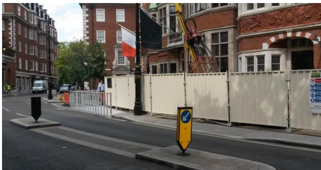
Image 1 - Rig inside hoarding
